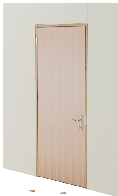
Leaf operation tested and gaps checked
