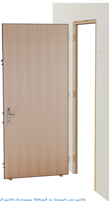
Leaf with hinges fitted is lined up with hinge recesses in frame using wedges
