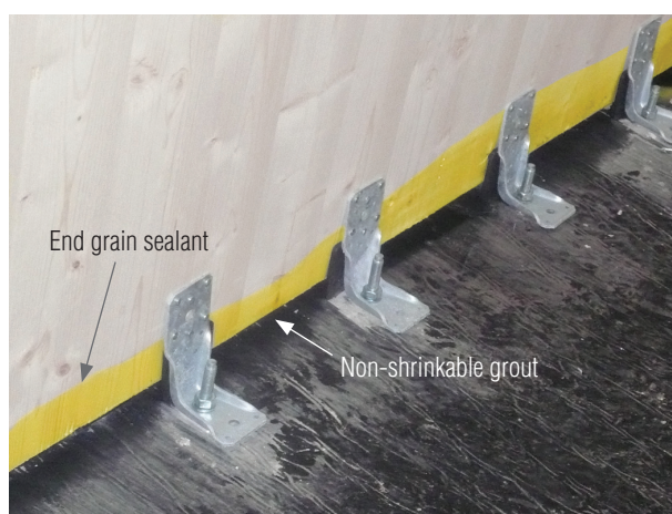
Fig 2.12 Standard fixing bracket to CLT (for option 1 in Fig 2.3)
