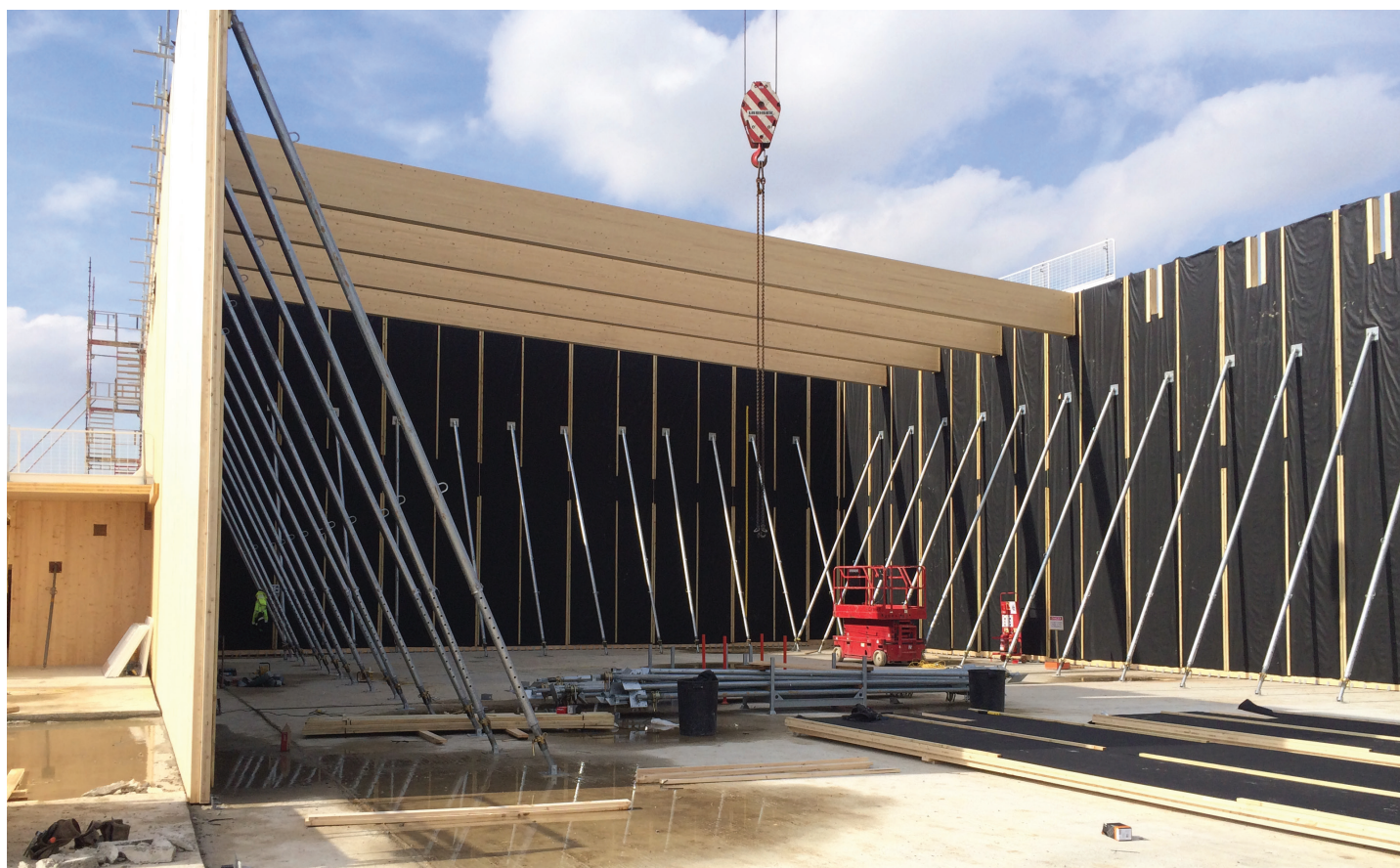
Fig 1 Temporary erection bracing and weather protection of CLT during erection
