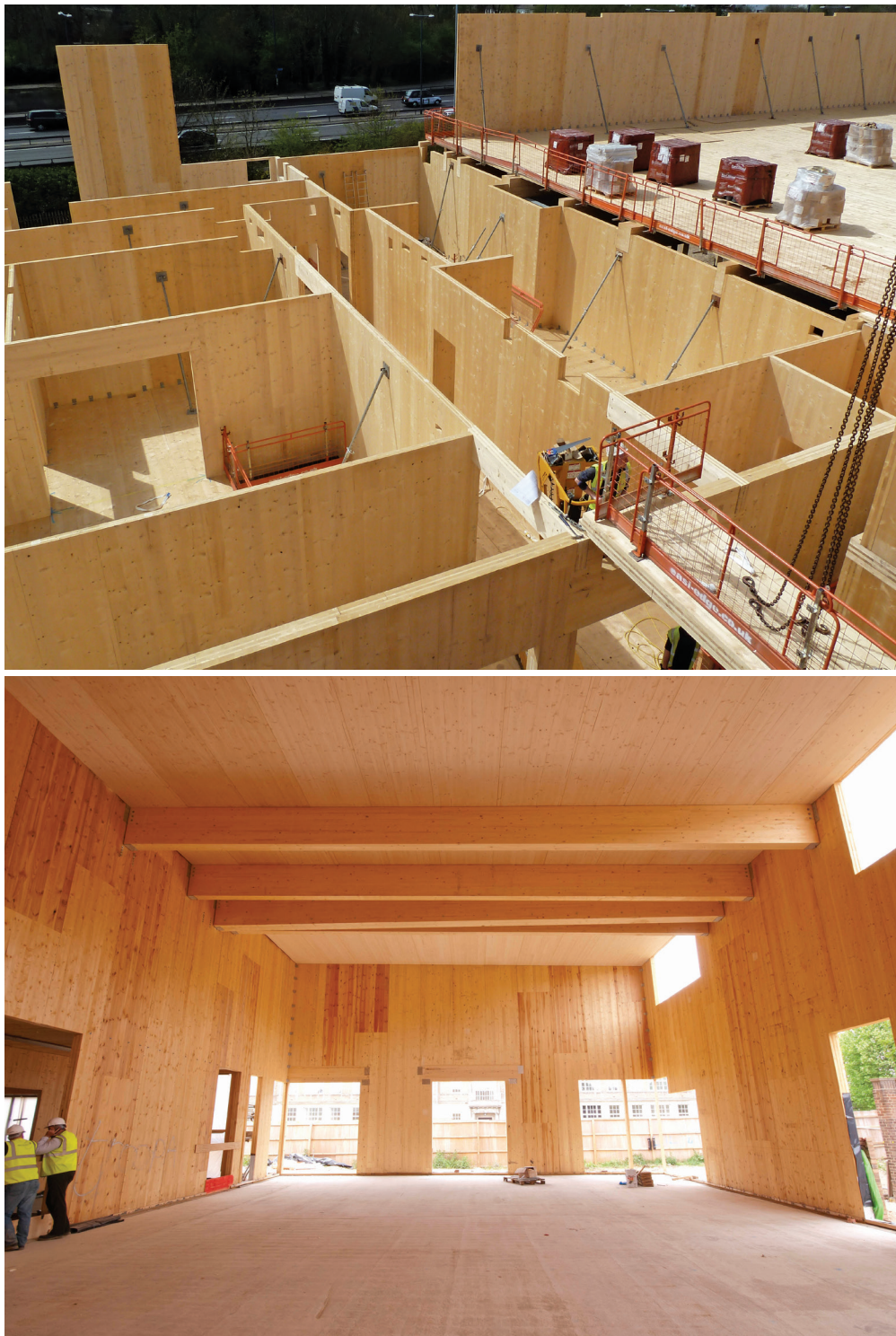
Fig 2 CLT panels during erection
