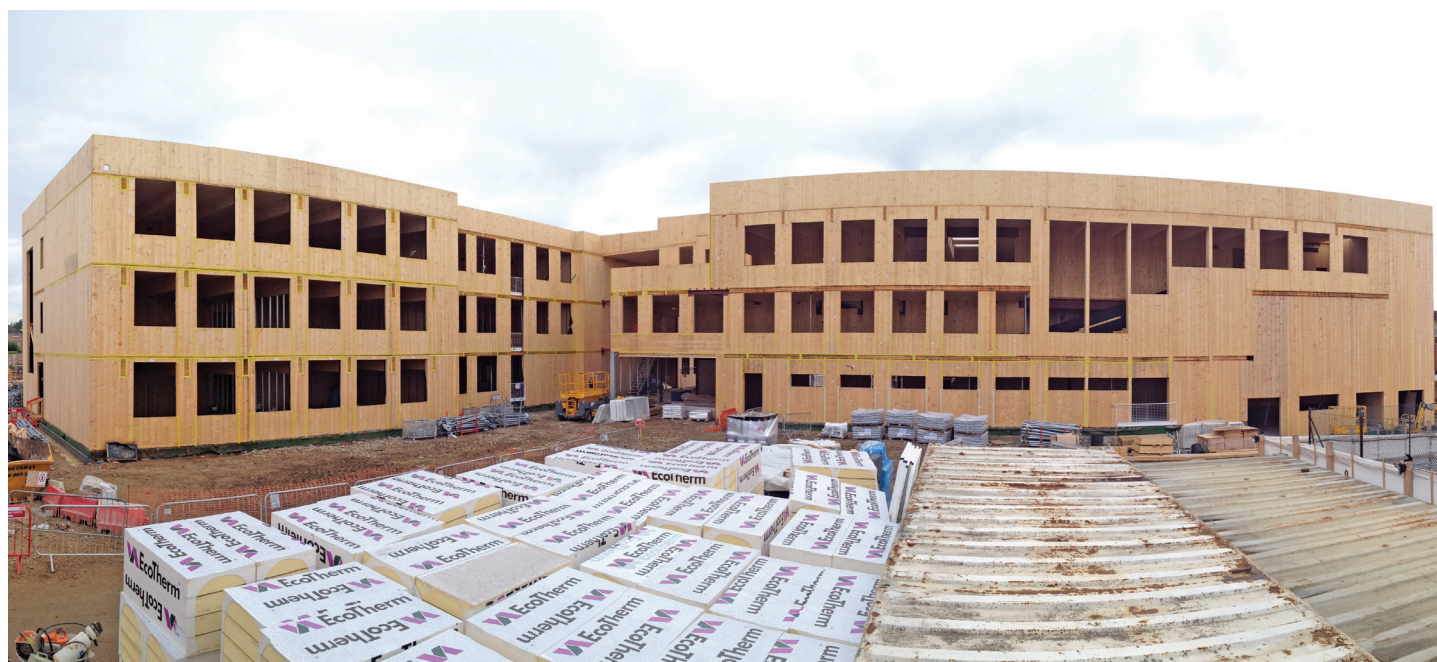
Fig 4 CLT structure during construction before cladding and insulation is installed
