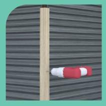
5) Finish cladding area by using angle trim, secure using coloured screws, please ensure you use countersink drill bit supplied in order to pre drill holes.
